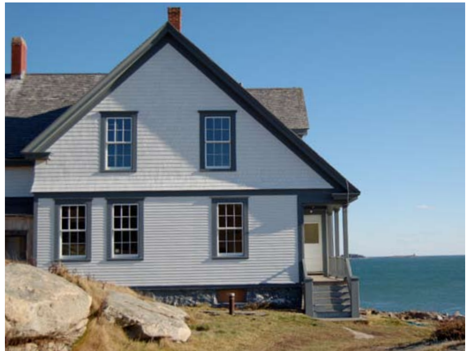
The Keeper's House at Whitehead Light Station
