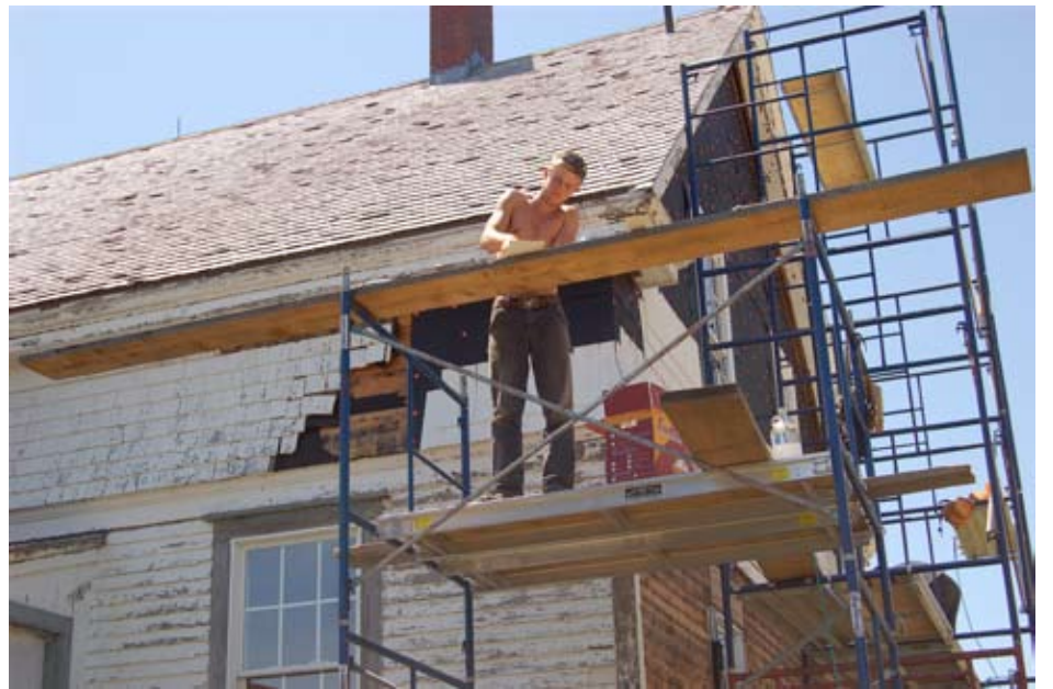
Off with the old shingles and on with the new
