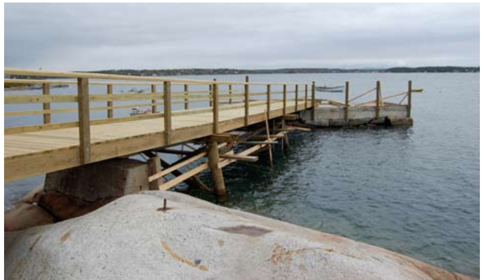
The new pier at Whitehead Island partially completed
